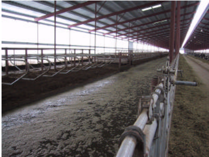
Free Stall Flush System - Flushing Feed Lane
