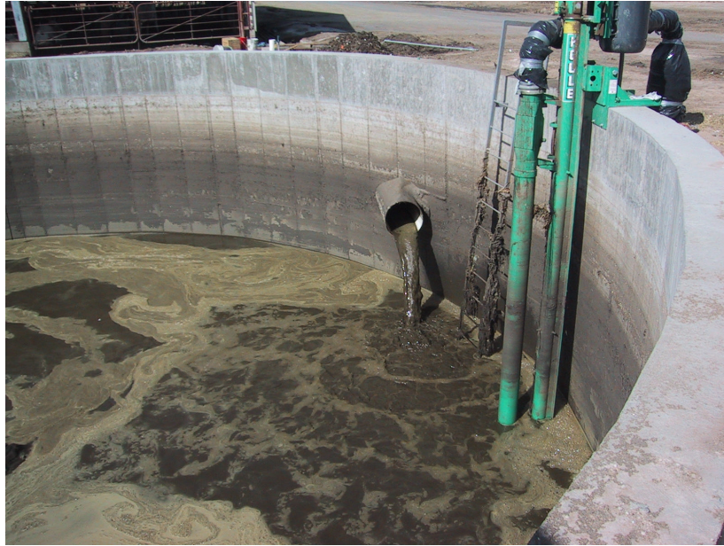
Typical Manure Sump with Chopper Pump
